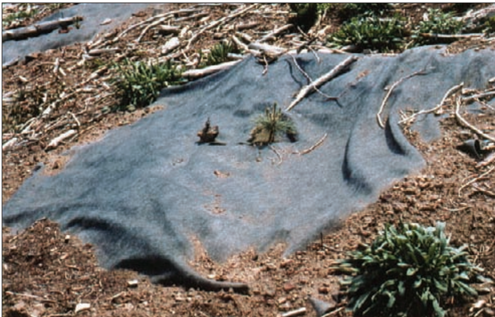
Figure 15—A 10- by 10-ft polyester mulch mat on a hillside with all sides tucked in.
