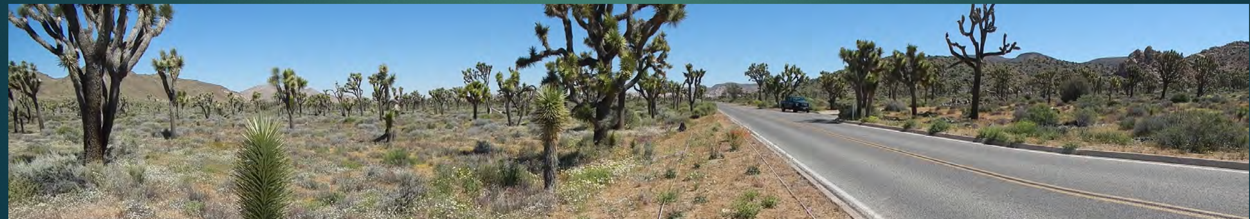
Roadside Outplanting and Vertical Mulching, Joshua Tree National Park
